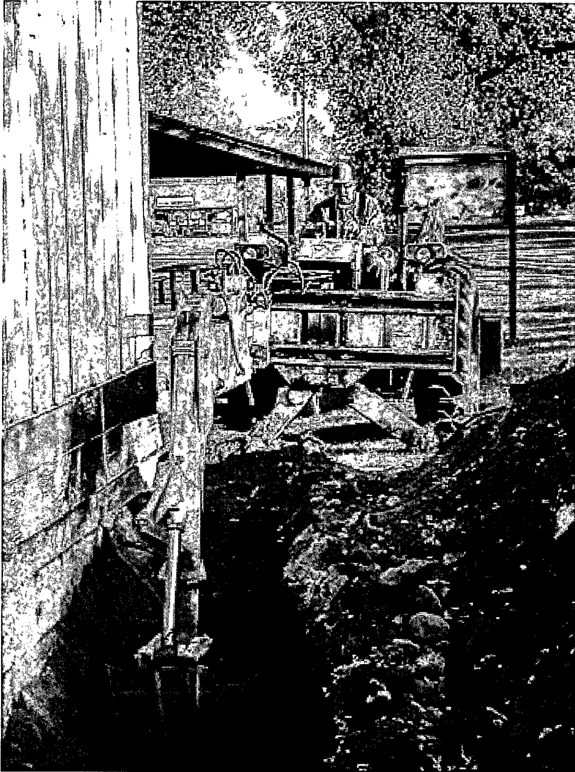
Figure 25. Historic Depot Excavation of eastside of depot foundation for stablization work.
