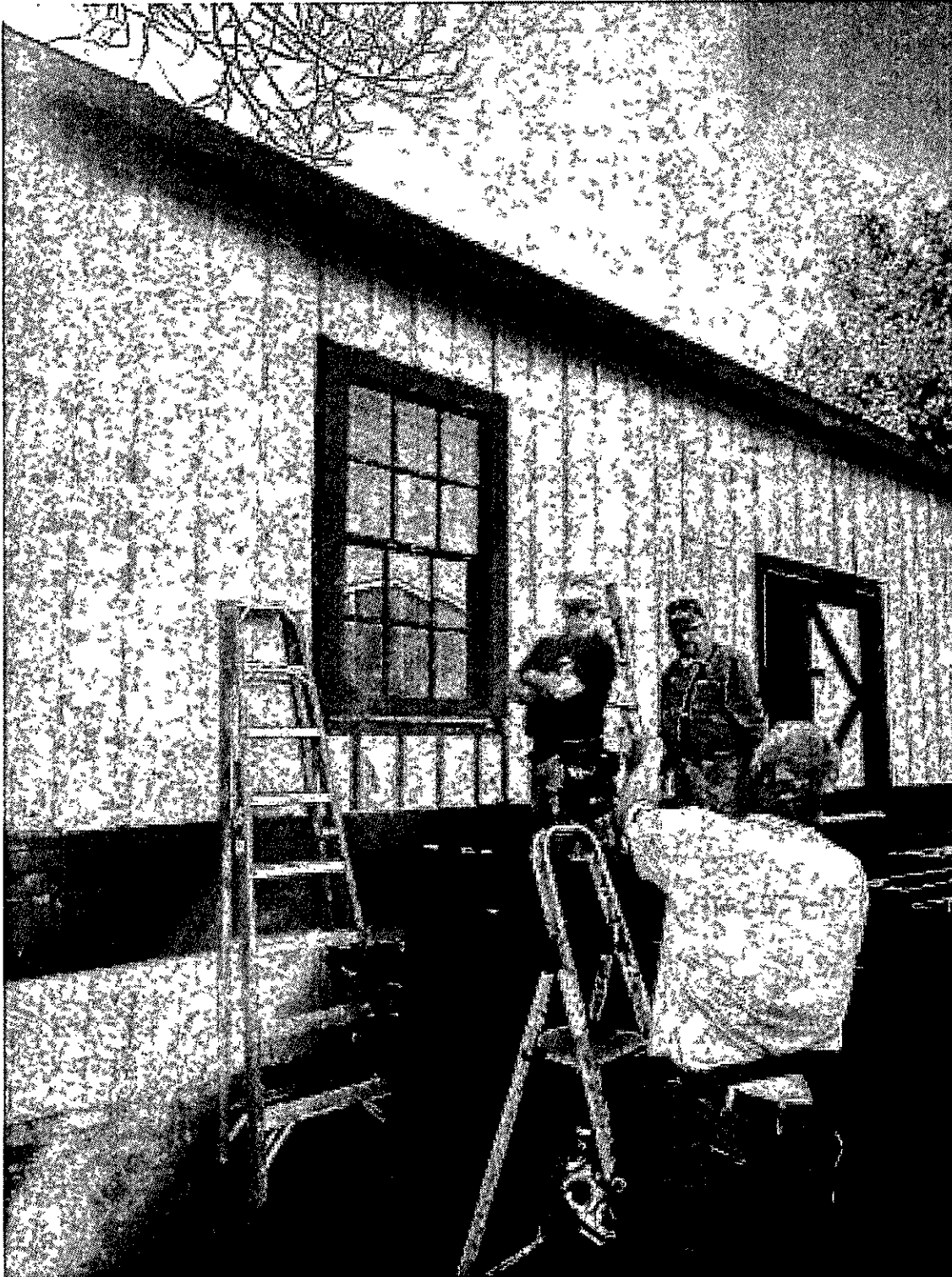
Figure 24. Historic Depot. Installation of hand-crafted bottle green painted windows on Finlayson's Northern Pacific Combination Depot.
