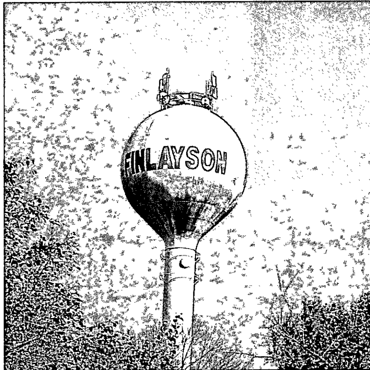
Figure 1. Finlayson Water Tower at School Street N & Water Tower Avenue
